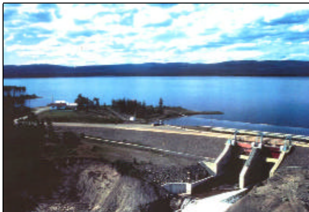
Photo 2-2 Skins Lake Spillway built to release water from the Nechako Reservoir into the Nechako River via the Murray/Cheslatta System.
