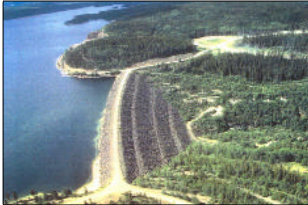
Photo 2-1 Kenney Rockfill dam constructed for the Kemano I Project to create the Nechako Reservoir.
